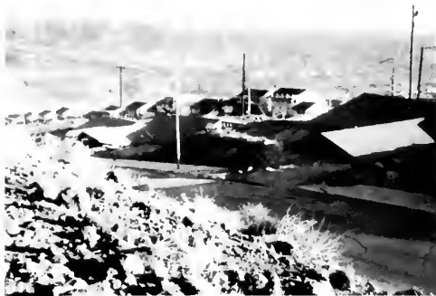
Photo 17. Shattered terrace deposits north of Walloby Avenue and about 122 m (400 feet) north of the Veterans fault (locality 48, plate 3). In the foreground, the roofs of houses under construction fell toward the north during the earthquake. Photo by F. Harold Weber, Jr.
